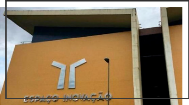
PST Guamá - CVACBA Building
